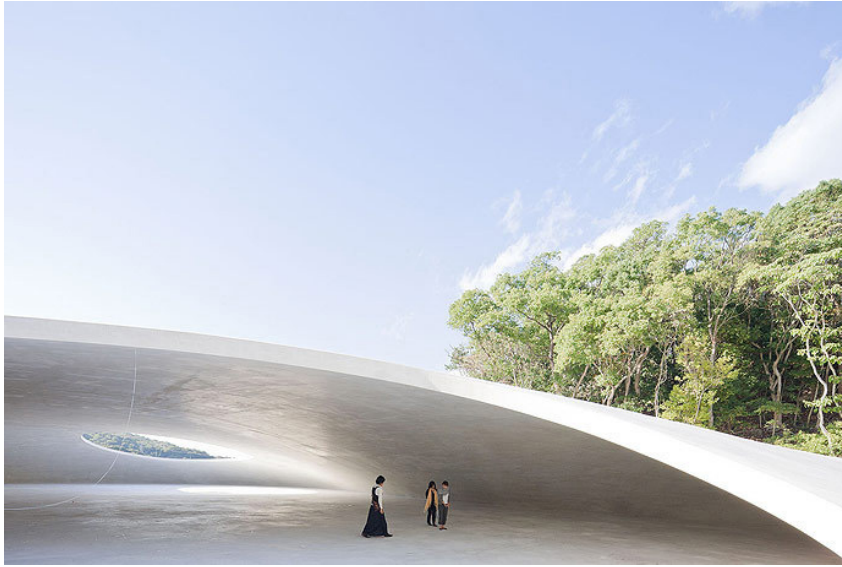
Fig. 8: interior view showing the thinness of the concrete shell
